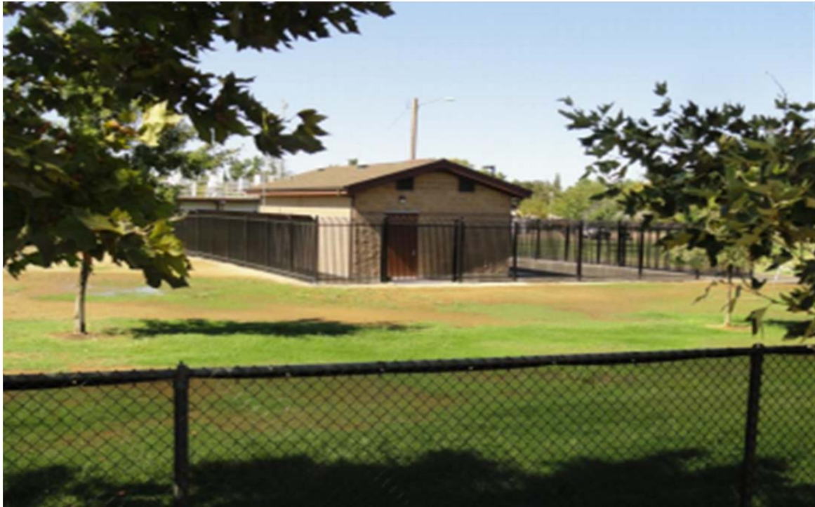
Del Paso Manor Water District Well #9, Constructed in 2010
